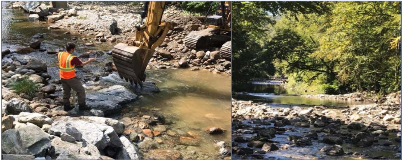
Figure 23. Staff from WRP and Harvey's Excavation working together to build a channel-spanning rock weir (left). A new pool complex for wild trout at the former Killooleet Dam site (right). Photos by the White River Partnership.
