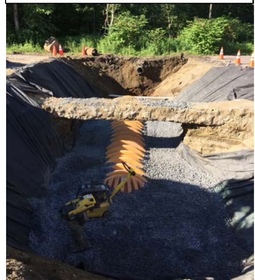
Figure 21. Stormcheck chamber to hold and slowly release stormwater runoff from the Warren School
